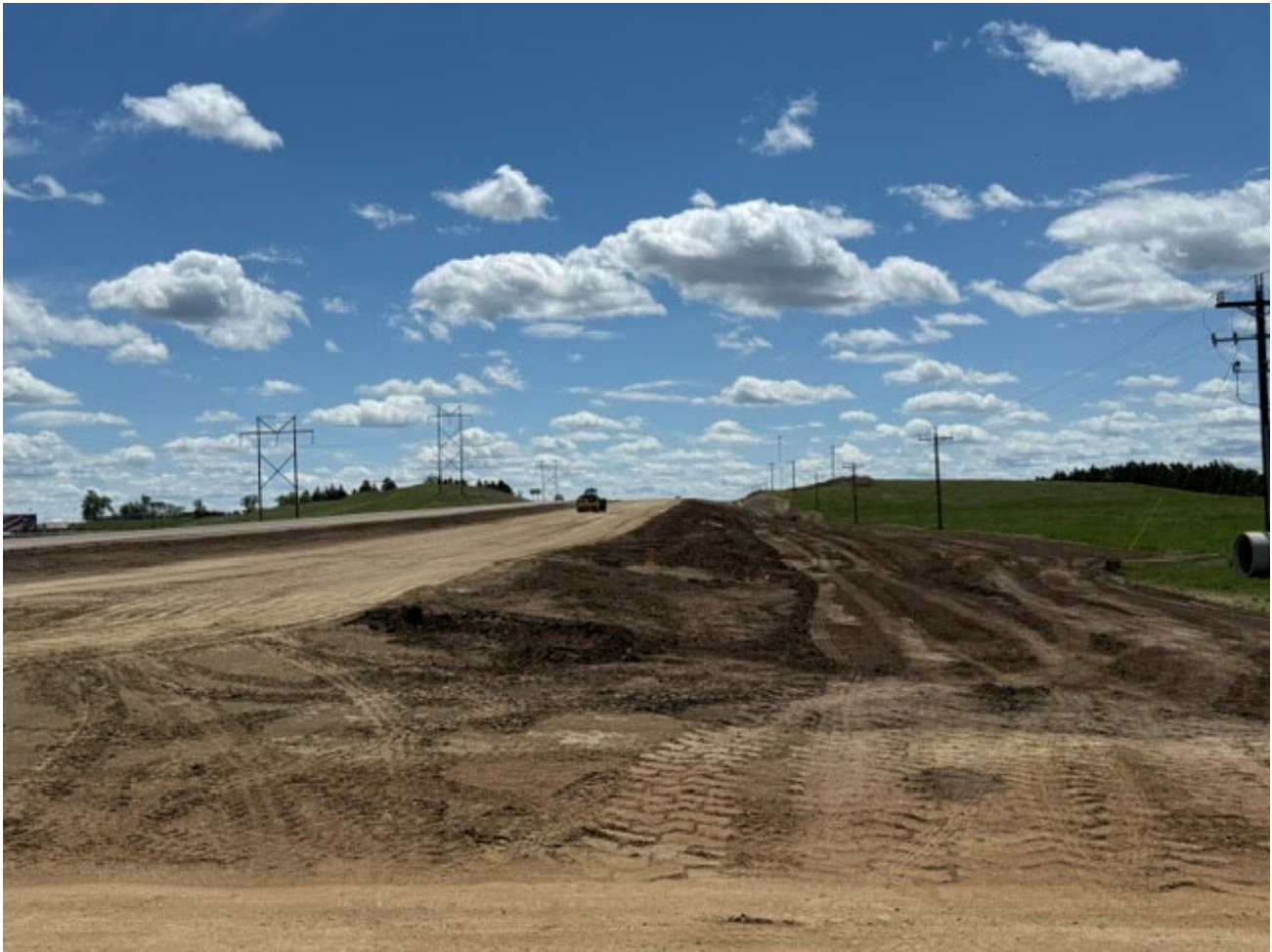
Roadway grading and future lane preparation along the U.S. 85 corridor.
