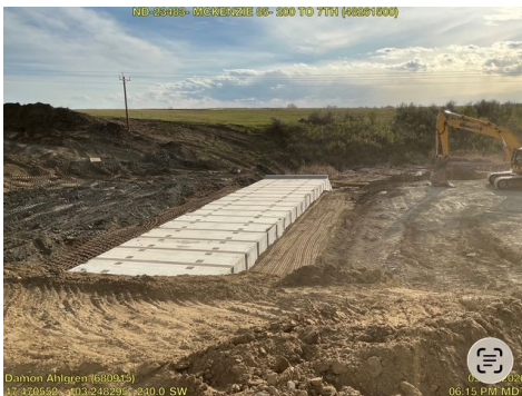
Box culvert sections placed at drainage crossing.
