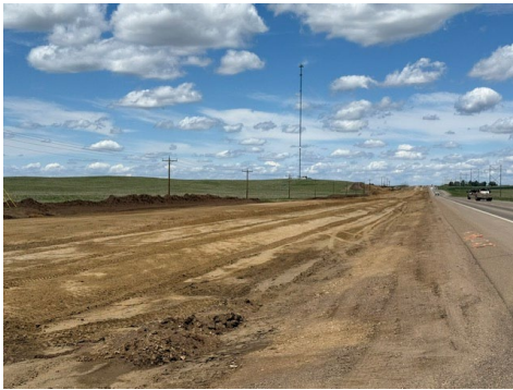
Roadway widening and embankment preparation.
