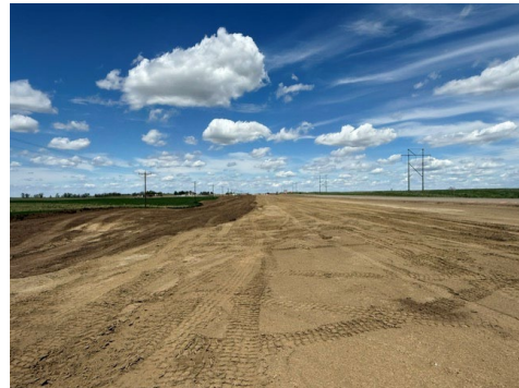
Corridor grading and roadbed preparation.
