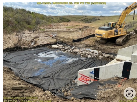
Drainage crossing preparation and erosion control.
