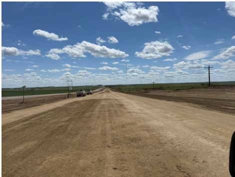
Grading and embankment work in open terrain.
