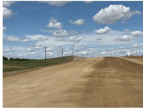
Prepared future roadway section.
