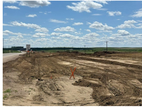
Subgrade and shoulder preparation along existing highway.
