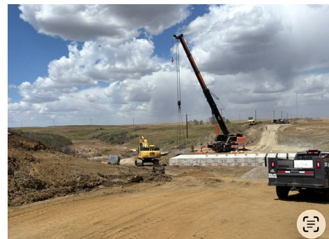
Crane operations setting culvert components.
