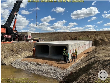
Completed box culvert installation with crews on site.
