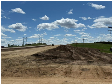
Roadway grading and future lane preparation.
