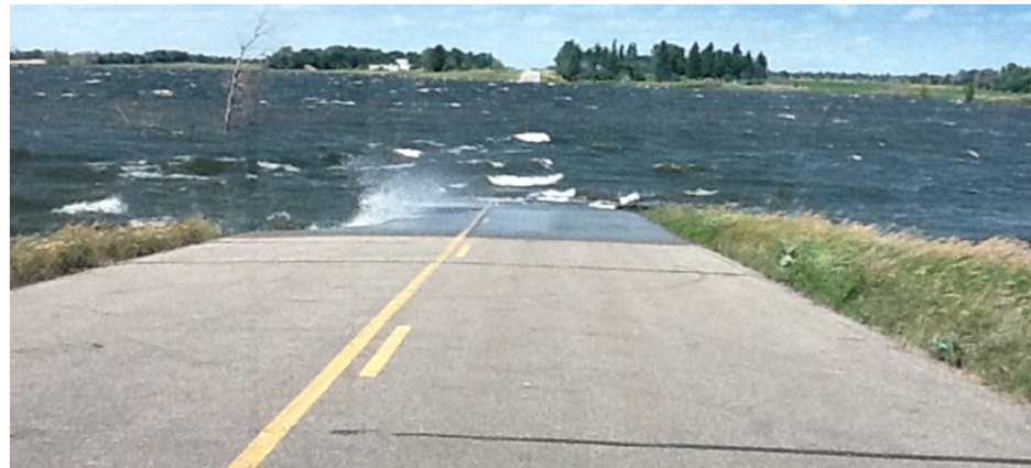
Lamoure County roadway
