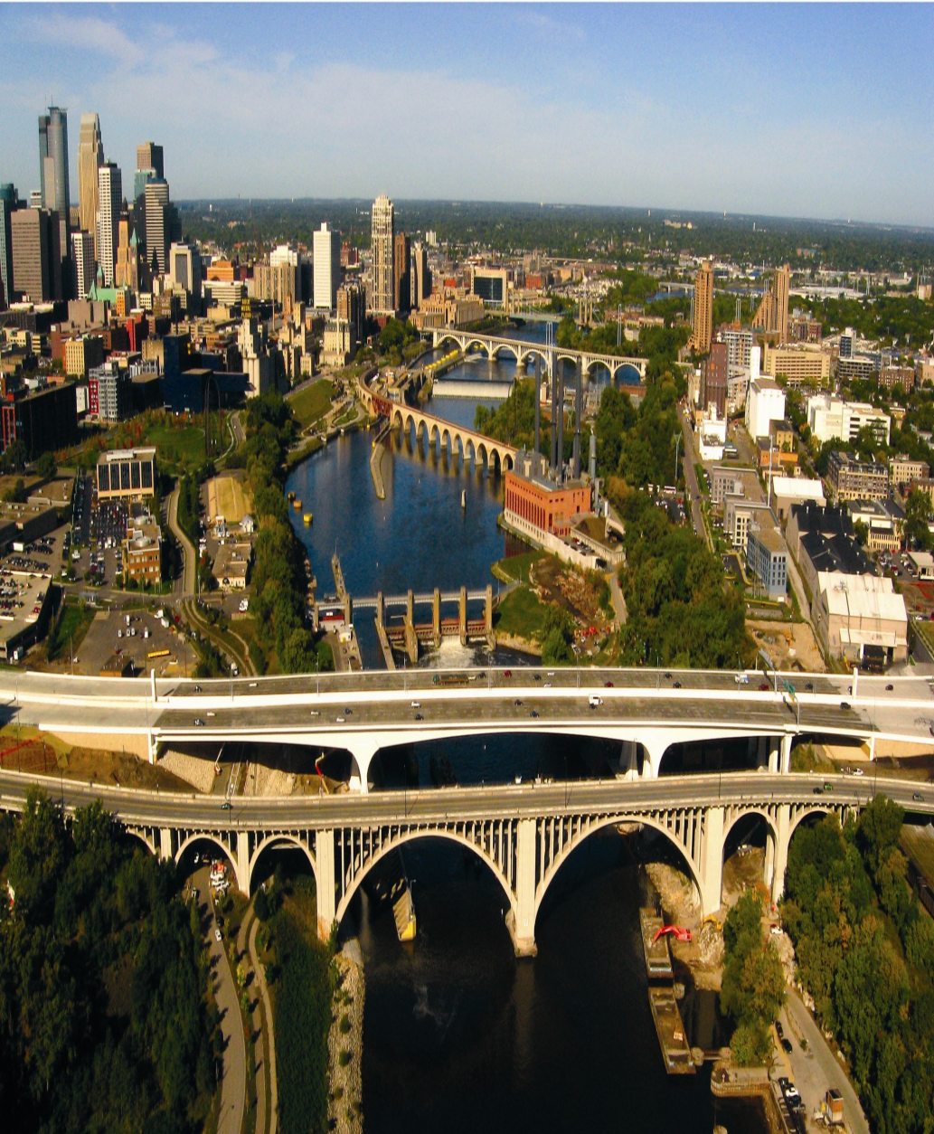
35-W Bridge Minneapolis, MN
